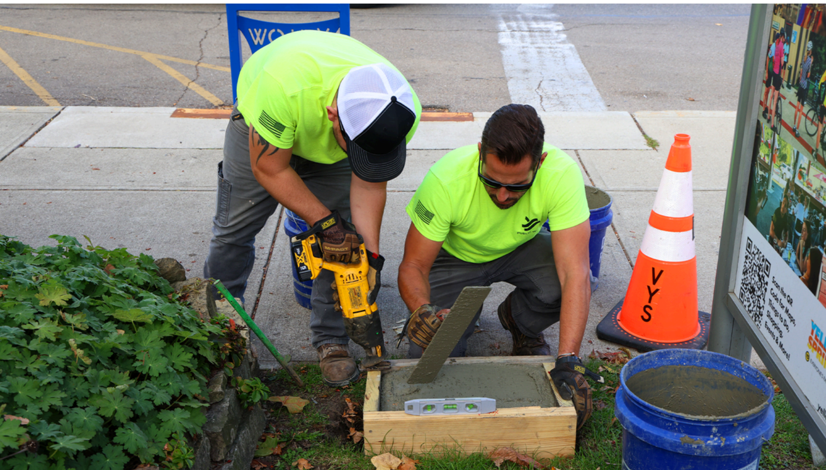
Village staff members Preston Harris and Tanner Bussey installing the new 365 Project Black history commemorative plaques
